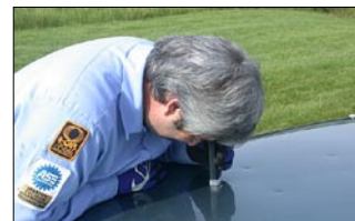
Figure 3—This technician is using a lighted magnifying tool to inspect the paint finish for micro-cracking in the hail damage.
